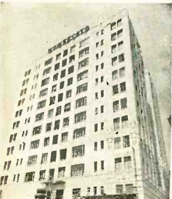
HOTEL - 120 Outlets - One Antenna - One Amplifier: The Montecito - 6650 Franklin, Hollywood, California.
